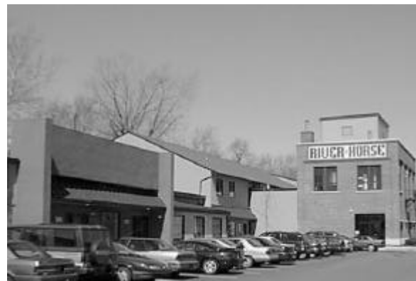
Former Oyster Cracker Factory was recently redeveloped in Lambertville, NJ, with federal funding assistance.
