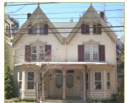
Gothic Revival, 1830—1890. Representing a transition from the classical styles to the Victorian age romantic styles, this style often includes bargeboard (gingerbread), steeply pitched, gabled roof lines, and sometimes pointed or arched windows.
