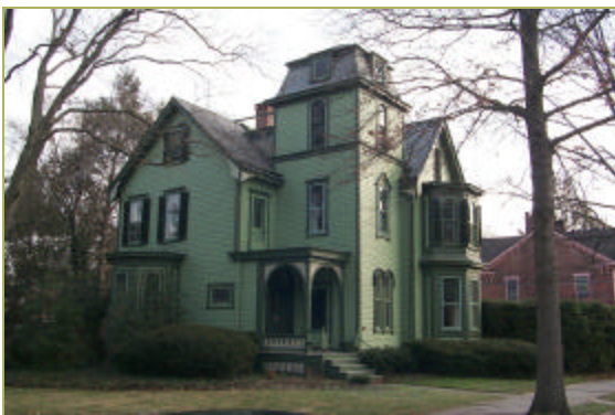
Italianate, 1835—1880. The Italianate style is the earliest form of Victorian architecture and typically includes long, vertical windows, heavily bracketed cornices and eaves, cupolas and porches.
